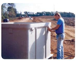
Attach nylon straps or chains to the lifting bolts.
